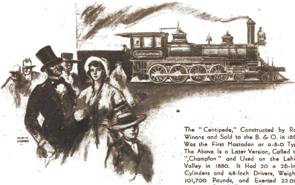
The "Centipede," Constructed by Ross Winans and Sold to the B. & O. in 1863, Was the First Mastodon or 4-8-0 Type. The Above Is a Later Version, Called the "Champton" and Used on the Lehigh Valley in 1880. It Had 20 x 26-Inch Cylinders and 48-Inch Drivers, Weighed 101,700 Pounds, and Exerted 23 000 Pounds Tractive Force
