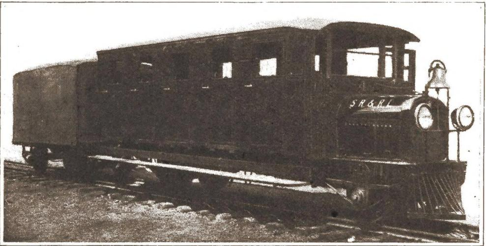
A Rail Bus Novelty—Passenger Coach with Baggage Trailer Truck. There Are Only Two of This Design in the World; Both Were Constructed by Sandy River Line for Its Exceptionally Narrow Tracks
