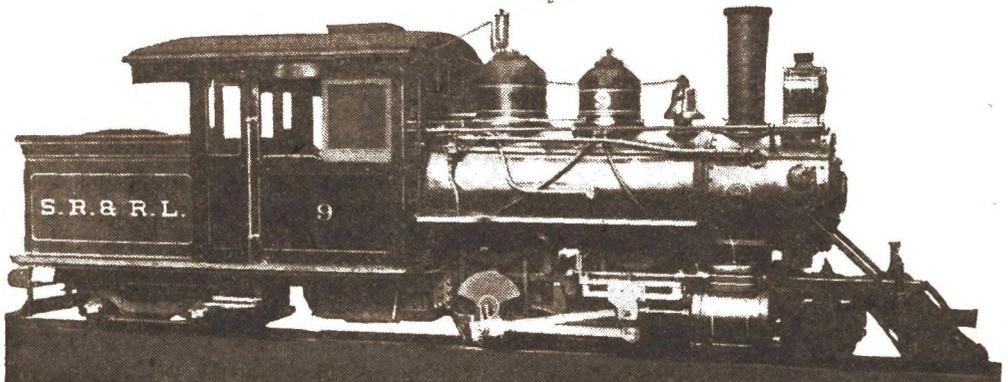
And Here's What a 2-Foot-Gauge Baldwin Passenger Locomotive Looks Like; Forney Type; 11 1/2 x 14-Inch Cylinders; 180 Pounds Boiler Pressure; 35-Inch Drivers; Total Weight, 56,750 Pounds
